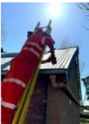
Images (Above,Left): Loose roof sheeting can be further damaged in a storm-our team had to make a temporary fix to this roof after a wind event
