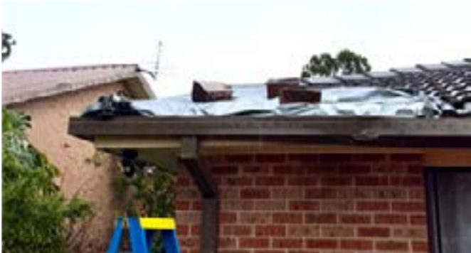
Images (Above,Left): Loose roof sheeting can be further damaged in a storm-our team had to make a temporary fix to this roof after a wind event
